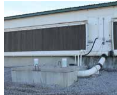
Barn fan and evaporative cooling pad.
